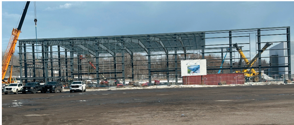
City of Thunder Bay Indoor Turf Facility Beverly Street
