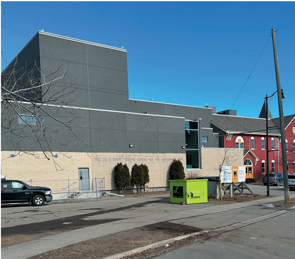
Magnus Theatre expansion and renovation
