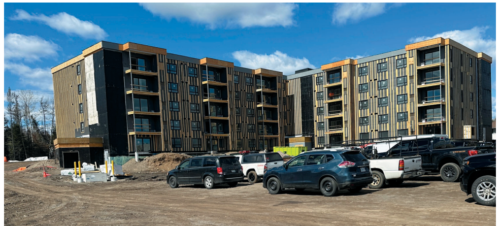
New apartment complex in the River Terrace area
